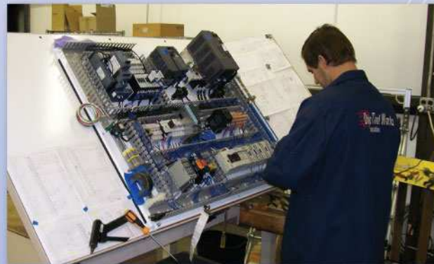
Electrical Panel Build
